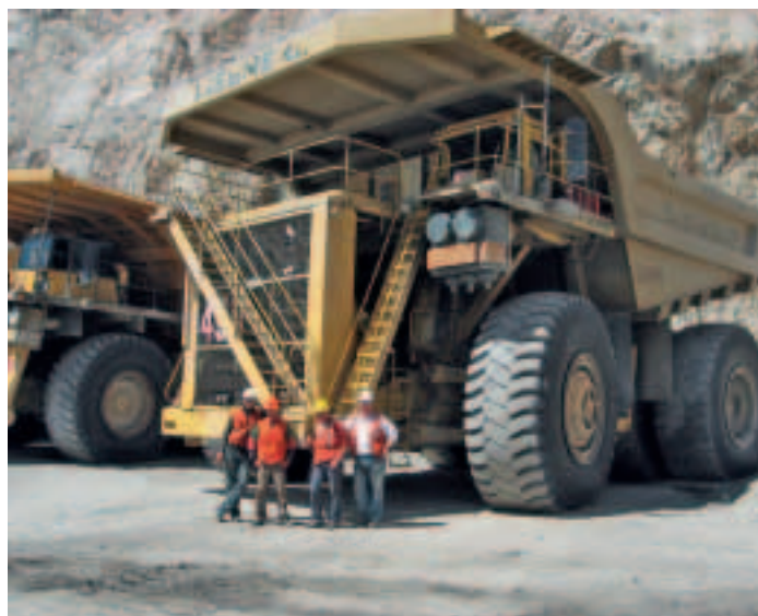
Installation and commissioning of an MTU Tier 4 Series 4000 pre-trial unit in a Liebherr haul truck in April 2009
